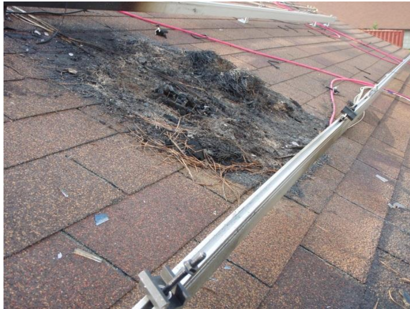
Figure 187 Roof after modules removed
