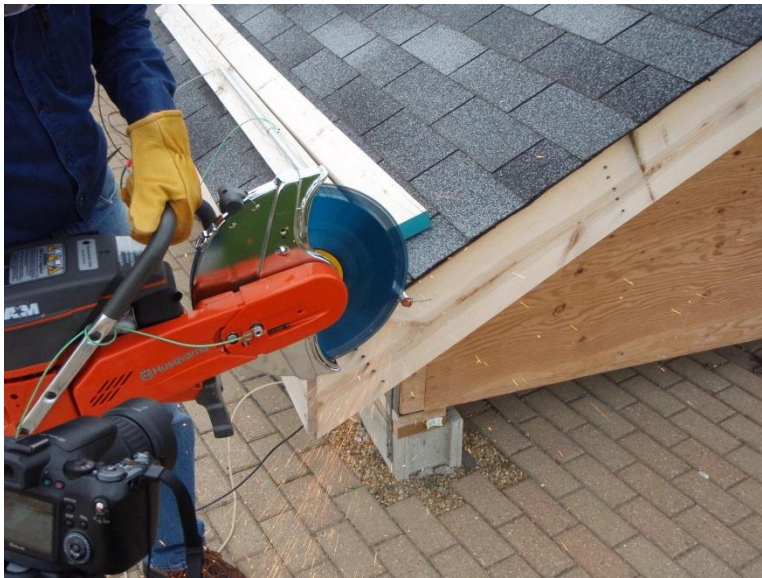
Figure 53 Rotary saw cutting through EMT
