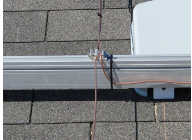
Figure 88 Grounding system for rails
