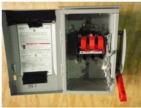
Figure 12 Switch S1 Open
