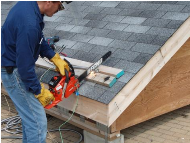
Figure 58 Cutting through flexible metal conduit
