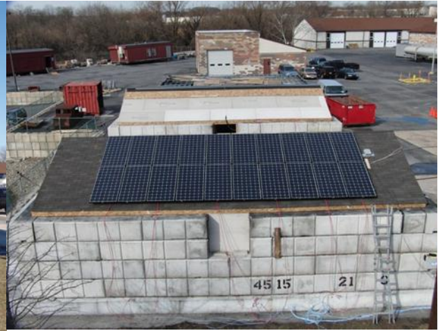
Figure 86 Framed module array from above
