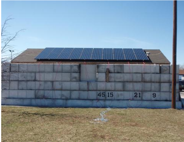
Figure 85 Completed framed module array
