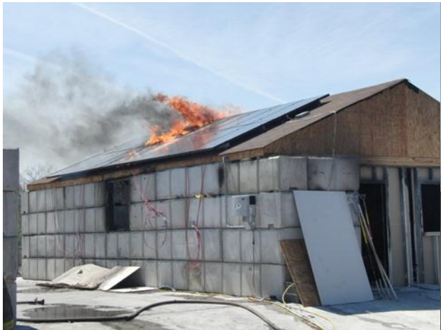
Figure 189 Ignited pine straw under modules
