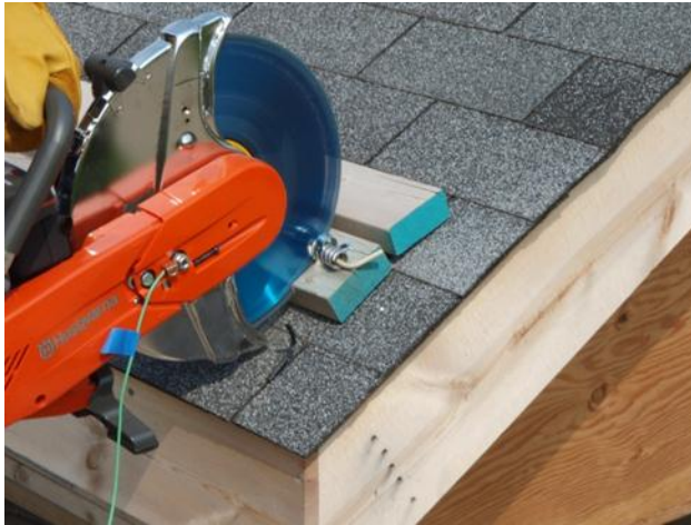
Figure 56 Cutting through flexible metal conduit
