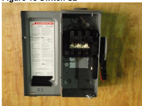
Figure 14 Switch S2 Open
