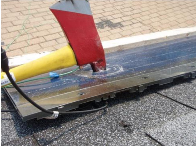
Figure 68 Axe pike damages PV shingle
