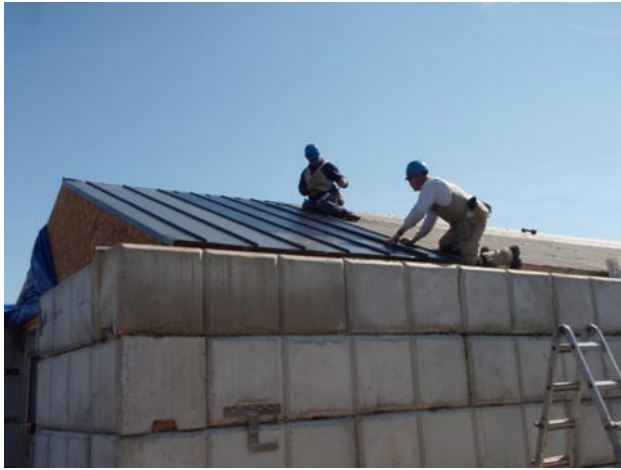
Figure 90 Installing laminates and metal roof
