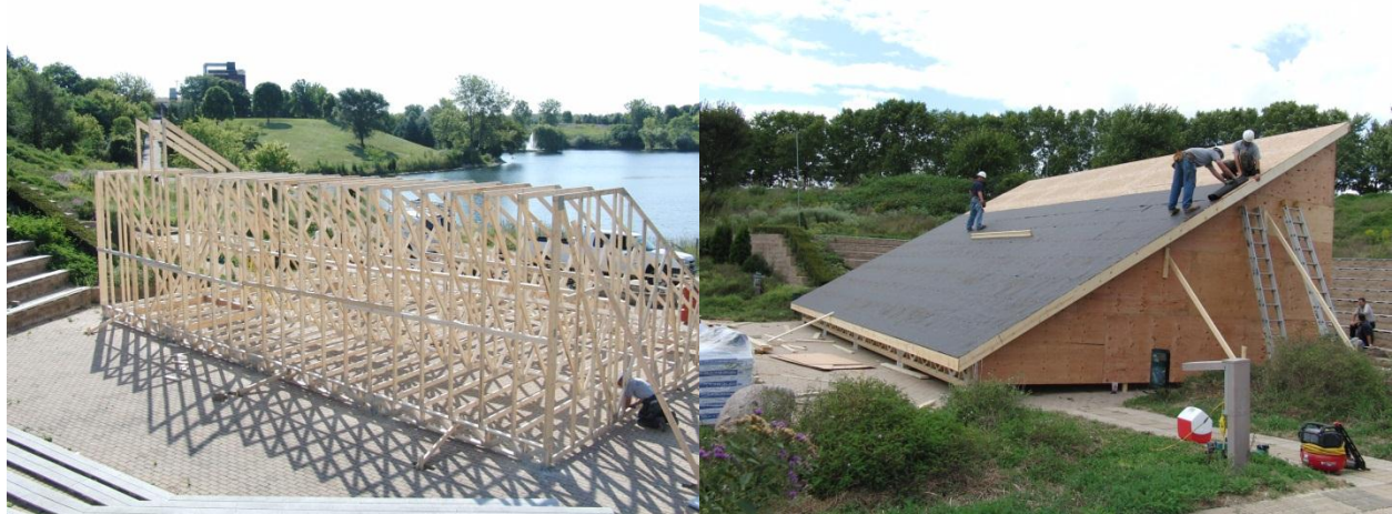
Figure 39 Construction of temporary PV test structure
