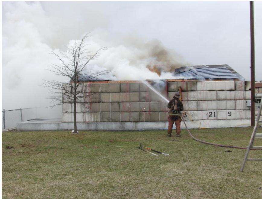
Figure 148 - Partial collapsed roof during extinguishment
