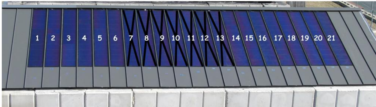
Figure 135 Roof diagram after fire: X = no power
