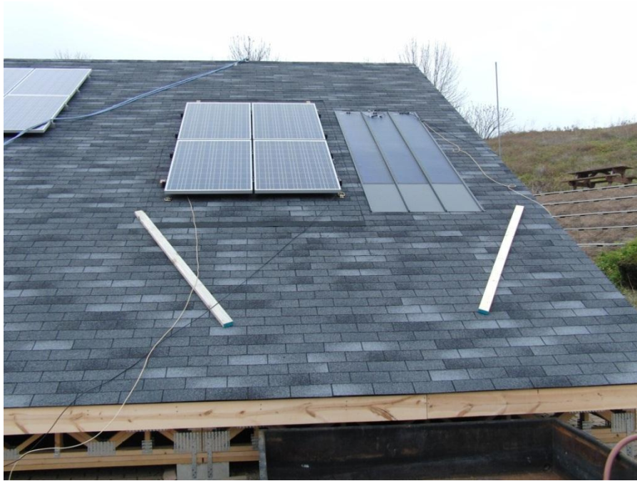
Figure 44 Test roof with four-framed module and three-laminate arrays
