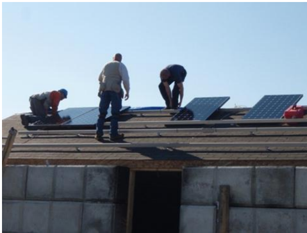
Figure 87 Installing framed modules
