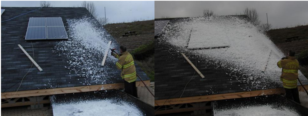
Figure 45 Applying Class A foam (1%) with compressed air foam system
